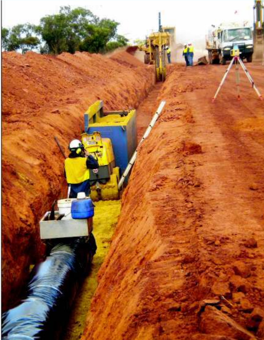
Pipe construction underway at the Karara mine site
